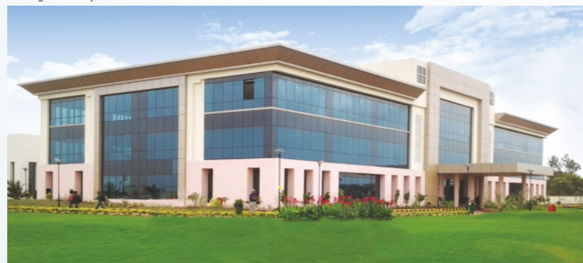
Switchgear Factory, Vadodara
